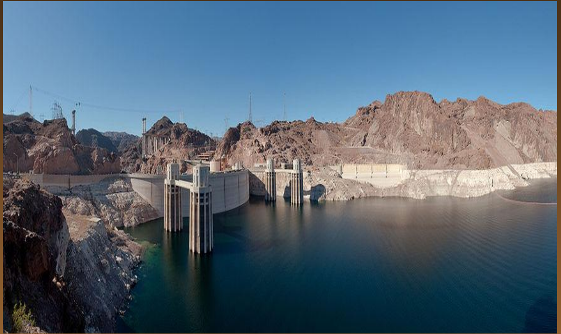
Hoover Dam – Colorado River
